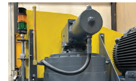
Mixer transmission lube station with pump and filter
