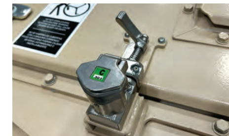
Hinged access door trapped key interlocks
