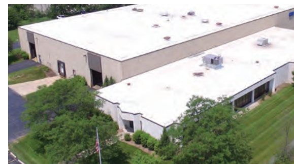
All under one roof at Mixer Systems headquarters: Design, engineering, manufacturing and a multi-million dollar parts inventory.
