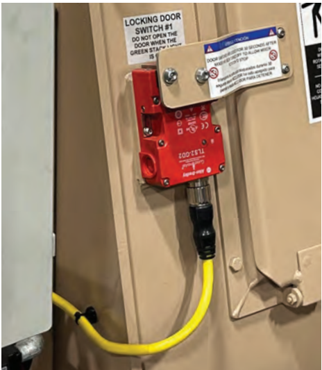
Access cover limit switch
